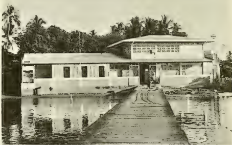
Fig. 3 - Frigorificos de Puntarenas, division of Borden Company, newest shrimp plant in Costa Rica. Puntarenas plants are small. Shrimp are sorted by hand, packed in cartons, and taken to a freezing plant.
