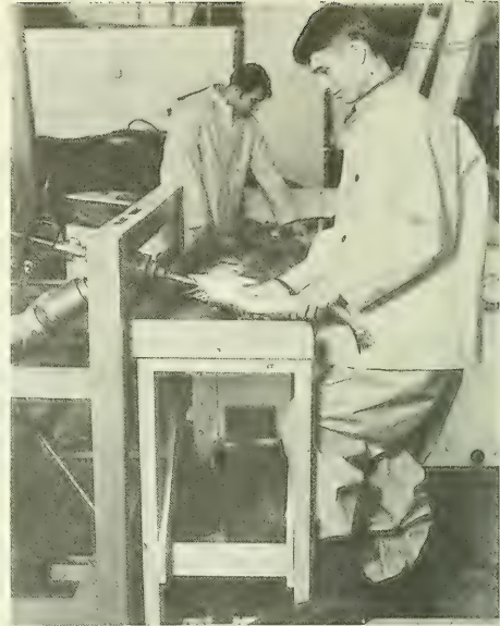
Fig. 1 - The vacuum evisceration technique.
