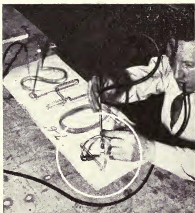
FIG. 57.—Sealing electrode to letter.
